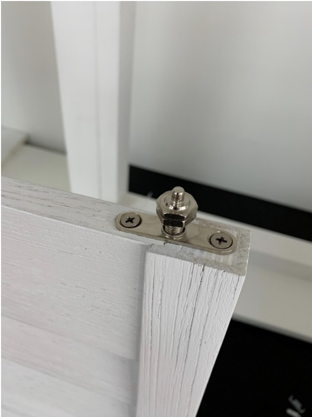
Bottom Pivot fixing on bottom of panel 1 and sometimes right panel.
