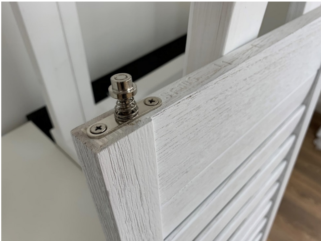
Spring loaded Top Pivot fixing at top panel 1 or very far right panel
