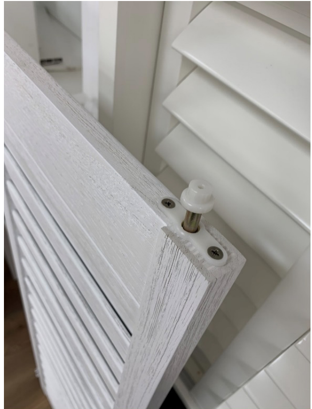
Spring loaded Bottom Guide on bottom of panels.
